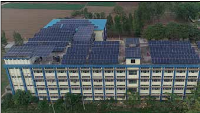
Chandigarh – Guru Gobind School | 200 kW Capacity
