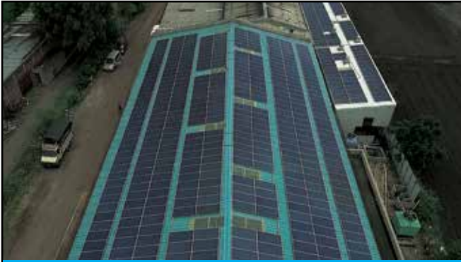
Ahmednagar – Katariya | 630 kW Capacity
